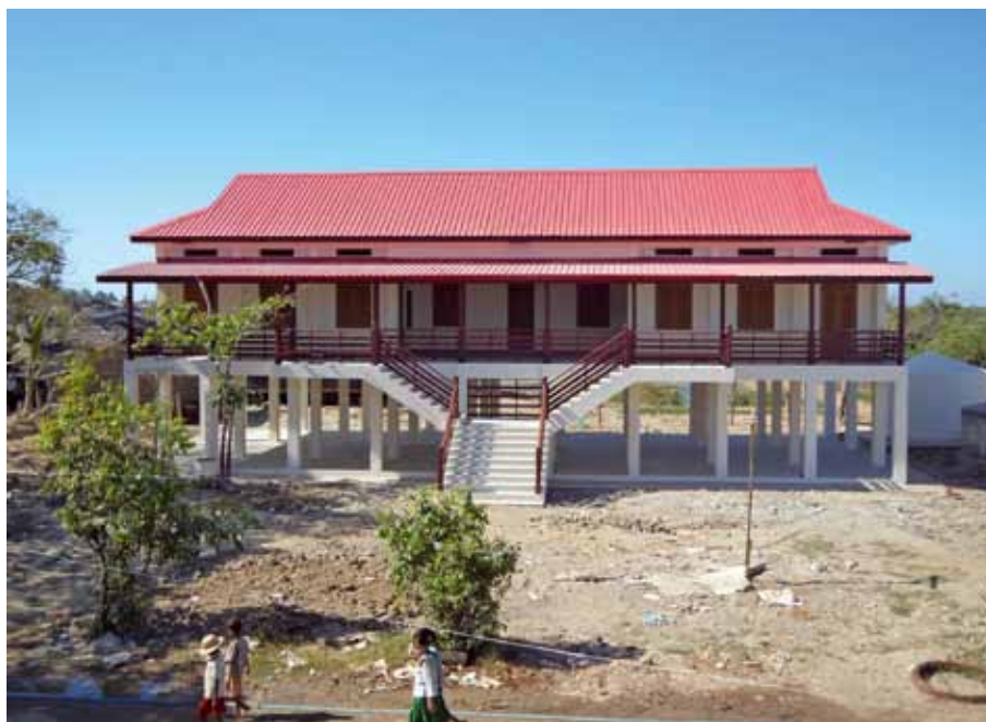
Cyclone-safe school in the Ayeyarwady Delta, of a similar type to the project co-financed by Liechtenstein
